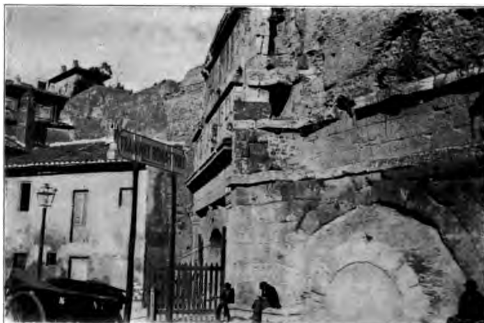
PORTA TIBURTINA, SHOWING THE CHANNELS OF MARCIA, TEPULA, AND JULIA GOING OVER IT. 2
